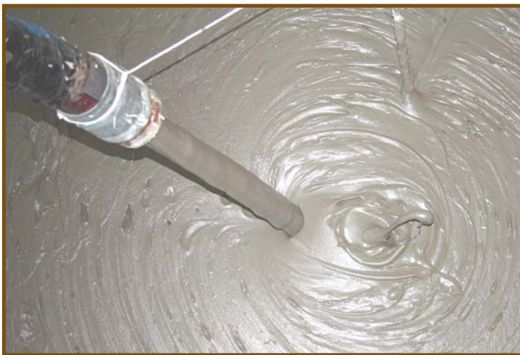
Pervious cellular lightweight concrete is a permeable, engineered material with a portland-cement base, containing small, open, air cells uniformly distributed throughout the concrete. The use of PCLWC in urban post-construction stormwater management practices provides improved runoff detention over granular pervious fill or lightweight aggregate materials.
