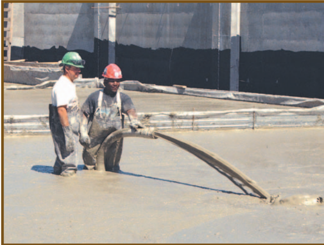
A highly fluid, self-leveling material, pervious cellular lightweight concrete (PCLWC) can be pumped long distances, with typical installation rates exceeding 100 cubic yards per hour.
