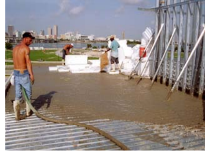
CLC Insulation on Steel Deck
