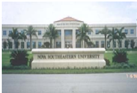
CLC Roof in USA
