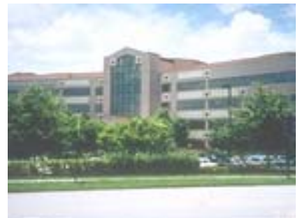
CLC Roof in USA
