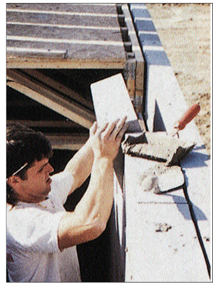
A special trowel is used when laying ACC block.
