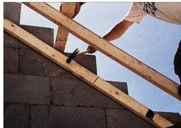
Autoclaved cellular concrete block can be nailed like wood.
