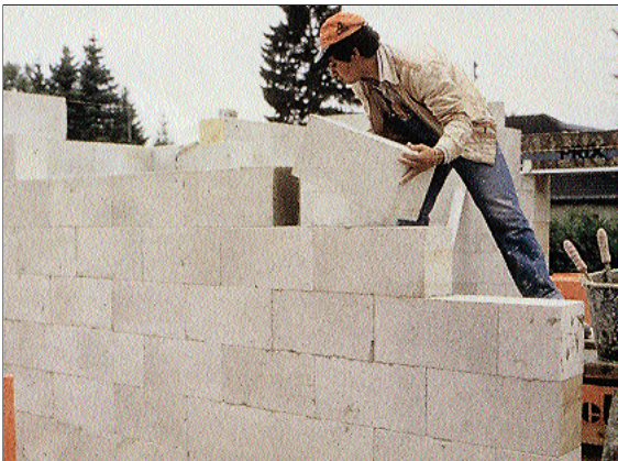
Wire-cut to precise dimensions, autoclaved aerated concrete block require only \frac{1}{8} inch of mortar at head and bed joints.
