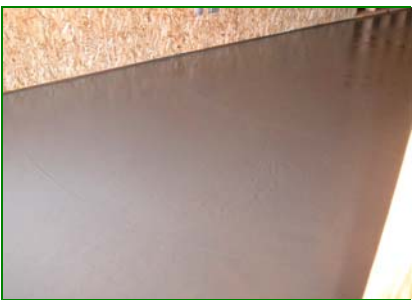
1000m 2 of Floor Finished in 1 Day
