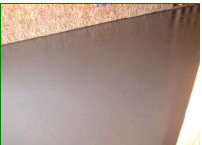
1000m 2 of Floor Finished in 1 Day
