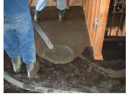
Self Leveling CLC Floor Insulation
